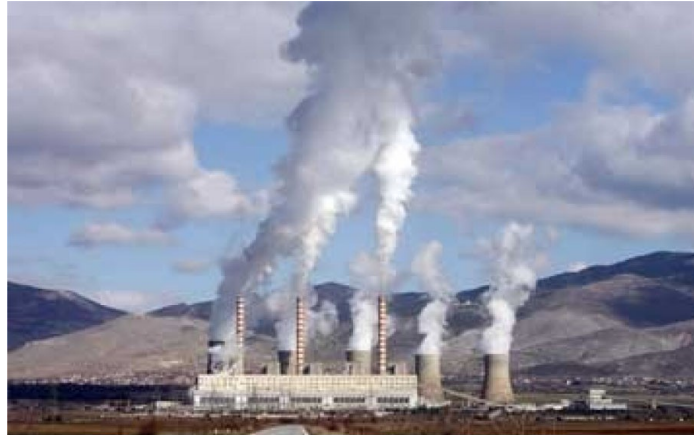
Figure 1. Photo of a real TPP (Kozani, Greece)
