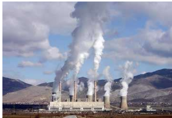
Real photo of a thermoelectric power plant
